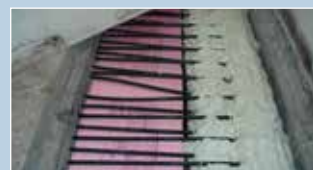
AFTER Insulated headers will eliminate condensation and frost, ensuring the mechanical system runs efficiently.
