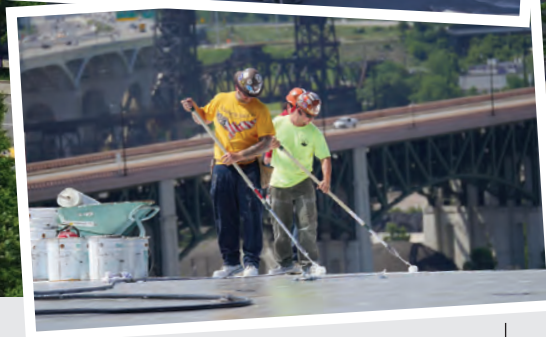
After the roof surface was cleaned, the restoration system was applied. The three-step process consists of a primer, a base coat with a fiberglass mat embedded in it, and a topcoat.
