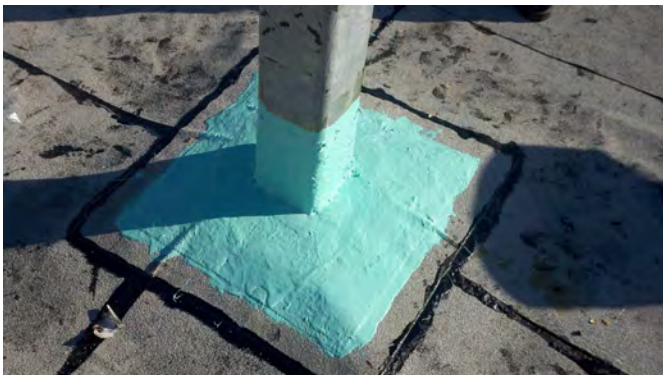
AlphaGuard as a flashing solution, is compatible with a variety of roofing systems.
