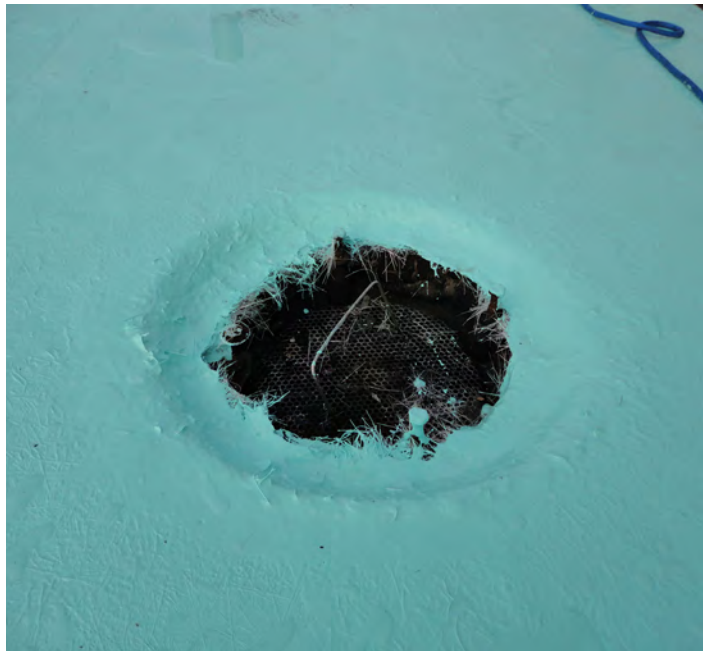
When flashing a drain, AlphaGuard will conform to the drain bowl, eliminating areas where water can penetrate.
