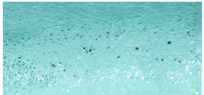
Fiberglass must be fully encapsulated in base coat without pin holes, voids, or openings.
