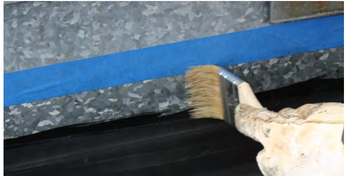
Prime all metal surfaces with M-Prime.
