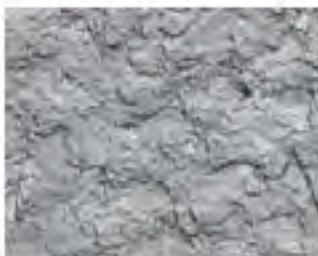
CSP 7 (Heavy Abrasive Blast)
