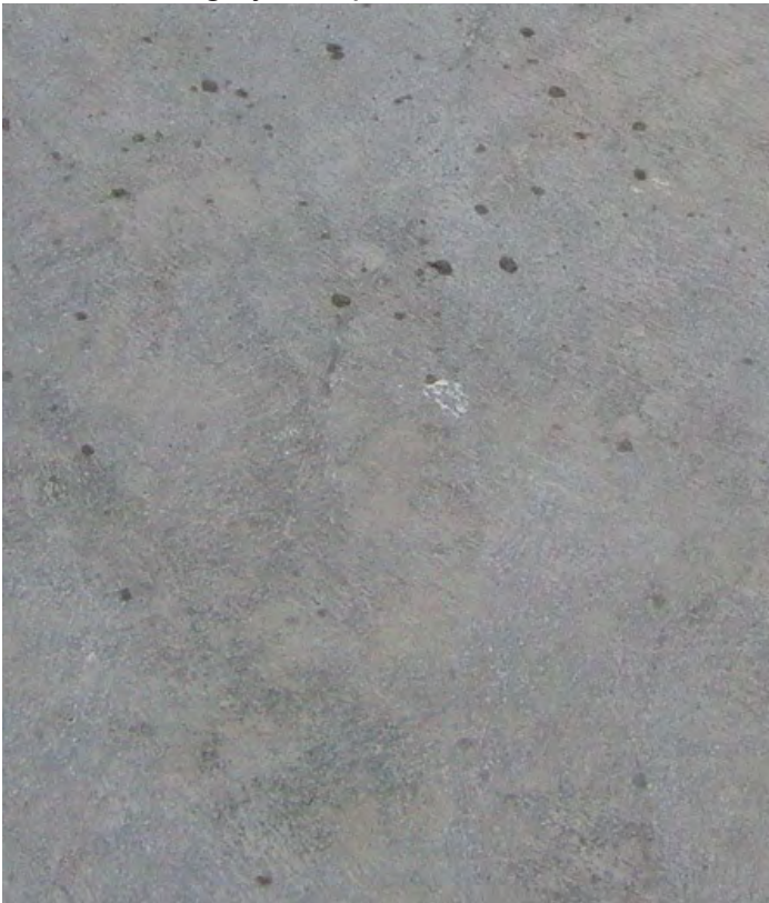
Properly prepared concrete substrate
