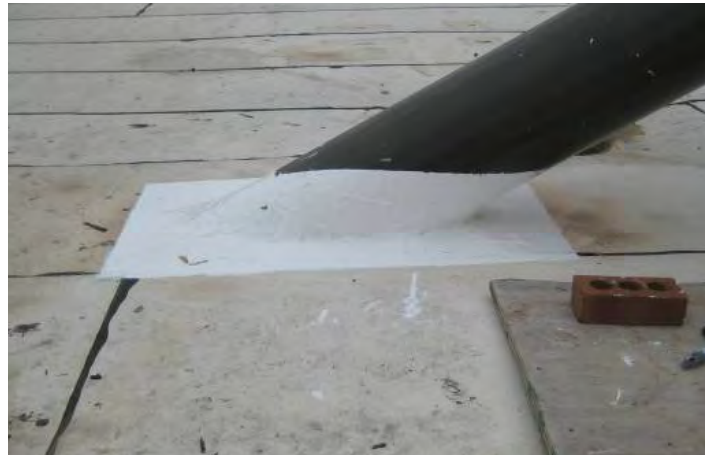
Penetrations on MB roof systems can be flashed with AlphaGuard as well.
